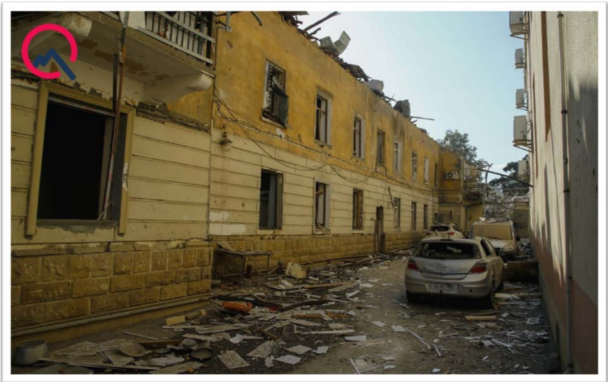
Photo 25: Damage inflicted upon the civilian infrastructure in the city of Ganja
