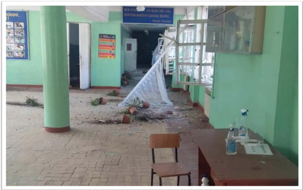
Photo 9: Damaged elementary school in the Ganja city
